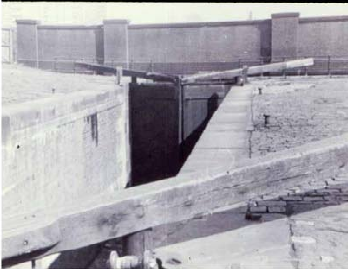
Lock 5 Head Gates - view towards Oldfield Road
