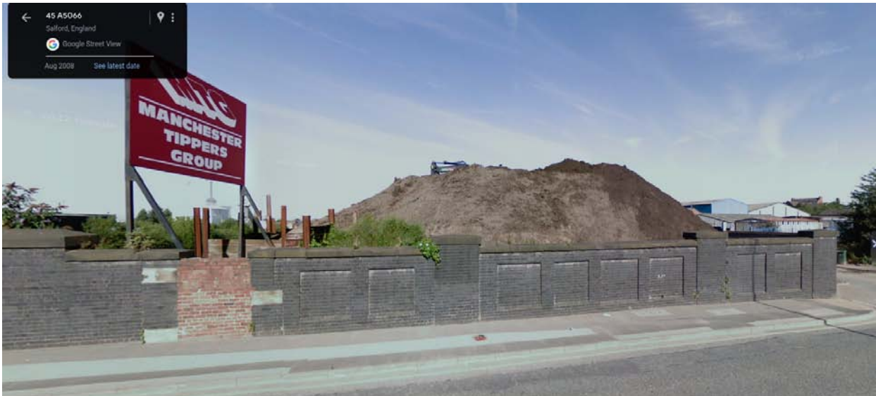
View taken in 2008 of the heritage canal bridge parapet showing the bricked up access to the original towpath (source: Google Street View).
