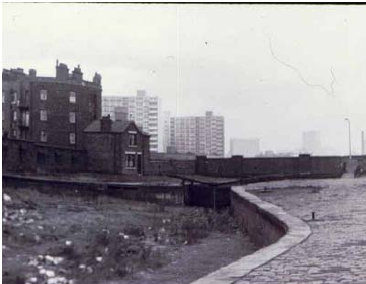
View of Lock 5 looking towards the Oldfield Road parapet with Oldfield Dwellings to the left.
